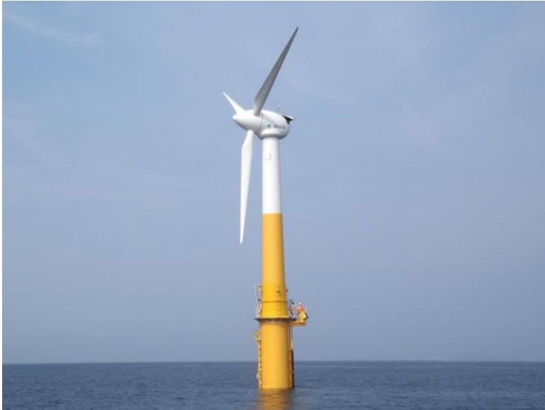
2 MW Goto island prototype
