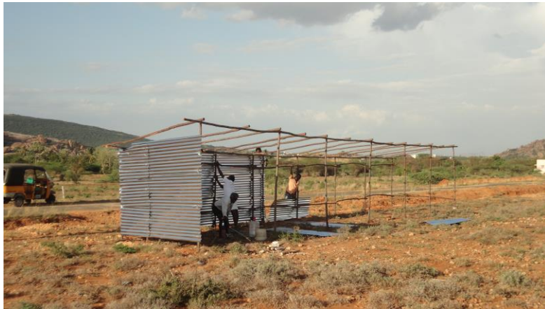
Temporary shed being erected
