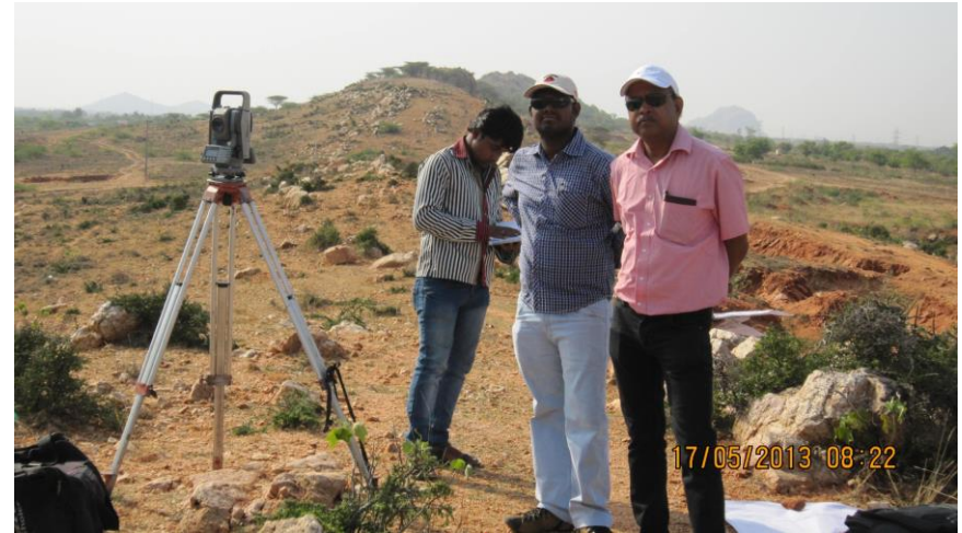
Surveyors in action
