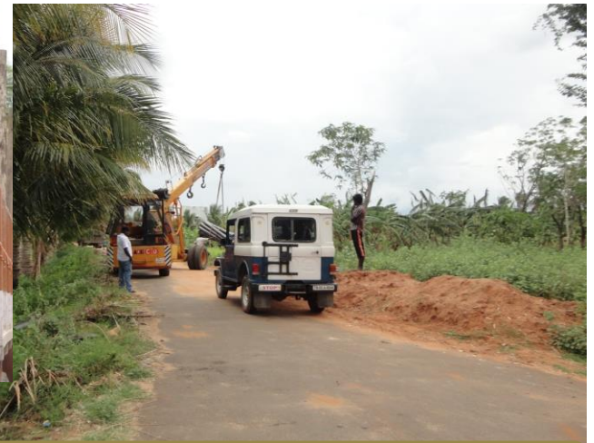
Unloading of water pipes near site
