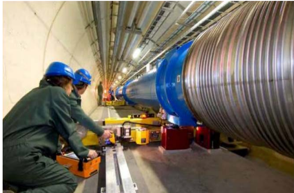
Indian made PMPS Jacks being installed in LHC
