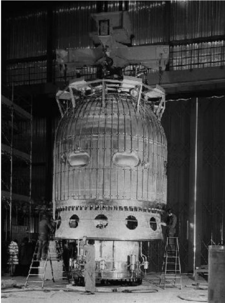
3.7 meter hydrogen bubble chamber at CERN, equipped with the largest superconducting magnet in the world.
