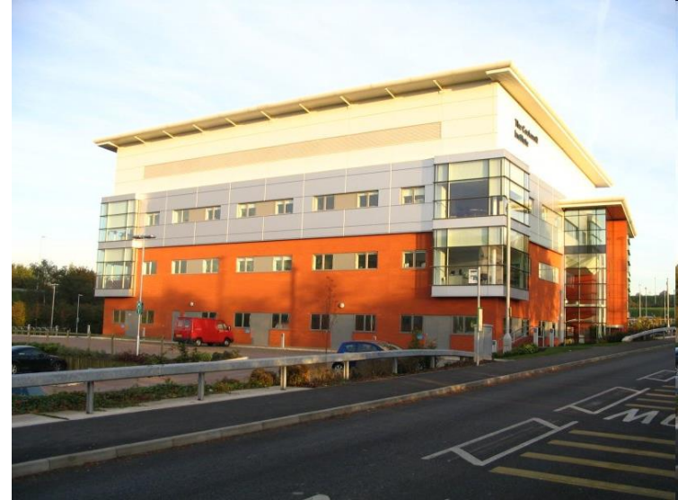
Cockcroft Institute Building at Daresbury
