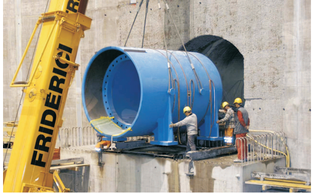
Figure 2: Installation of a part of the the ATLAS shielding in the UX15 cavern (a photo from the CERN Multimedia and Outreach Collection).
