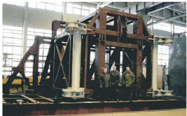
Figure 3: The frame of the blockhouse for the CMS forward shielding at the IHEP workshop (a photo from the IHEP Photo Gallery).
