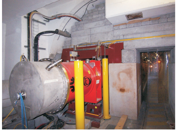
Figure 12: Machine background shielding in IR8, as installed at the IR1 side around the Q1 quadrupole (courtesy of D.Lacarrère).
