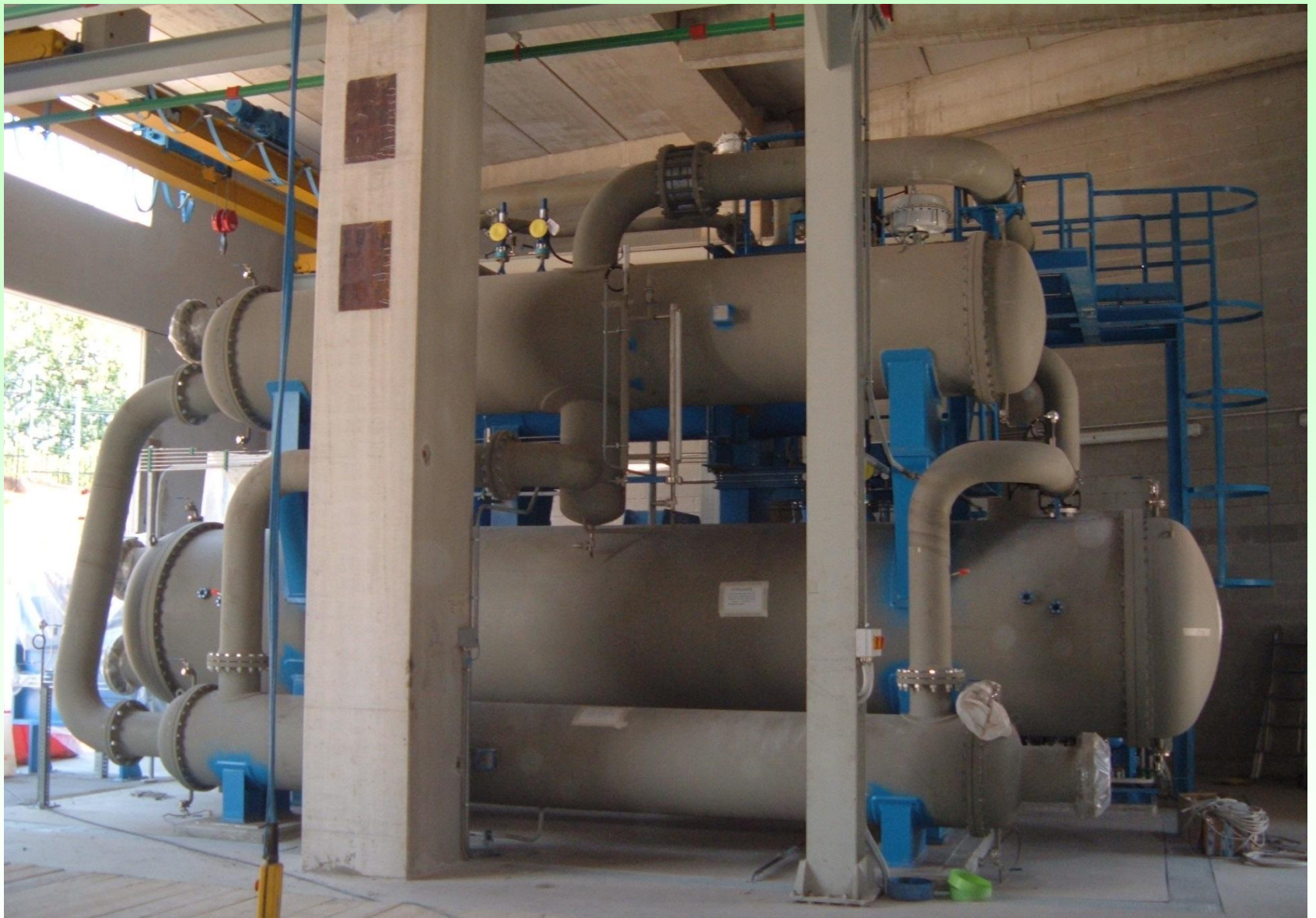
15 MW GROUND WATER HEAT PUMP WITH CENTRIFUGAL COMPRESSOR FOR A2A CANAVESE DISTRICT HEATING SYSTEM IN MILAN
