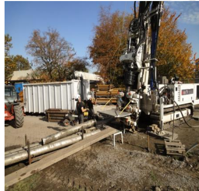
DTH water hammer makes for very fast drilling and excellent seismic noise source
