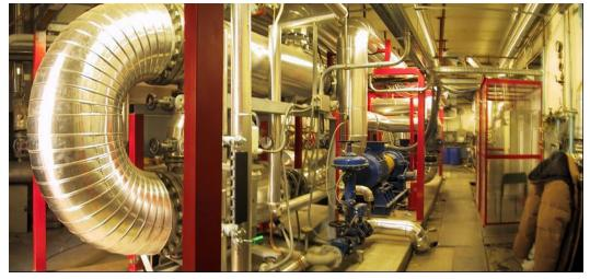
The **Thermal Energy Storage** (approx.  $1.000 \text{ m}^3$  each one) are used for reducing the usage of the boilers during the daily consumption-peaks  $\rightarrow$  **Optimization of the exploitation of the renewable and recovery sources**  $\rightarrow$  Decrease of methane use
