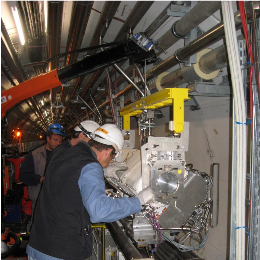
At end of crane boom
