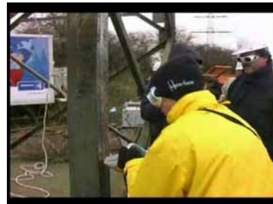
Laser cleaning with hand held 1.5 kW system (By CLEAN Laser Systems)
