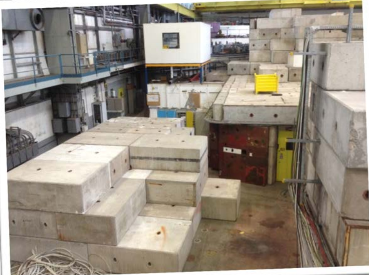
T7b area dismantled
