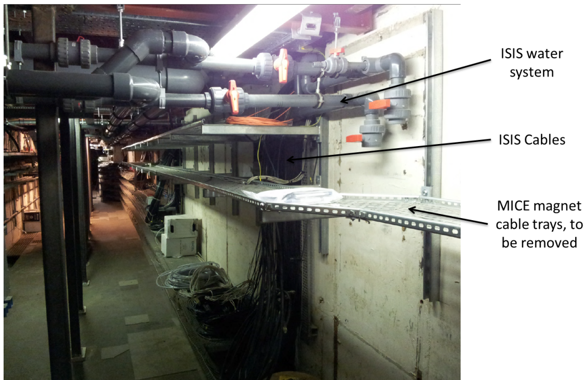
Figure 104: Existing services in the Trench, looking from West to East.
