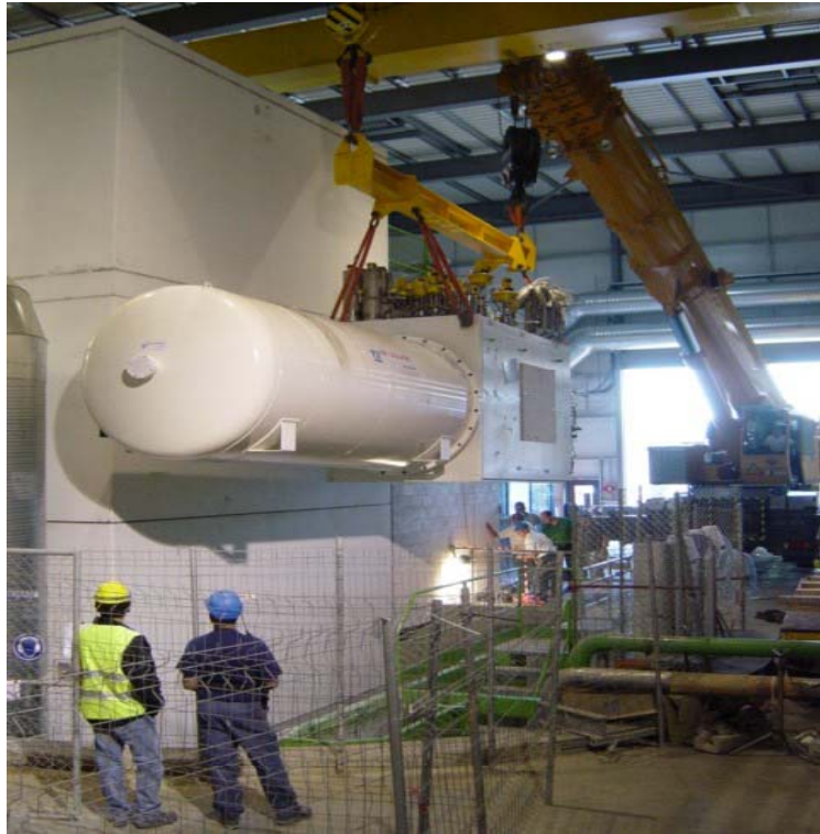
He Main Refrigerator: 6 kW @ 4.5 K
