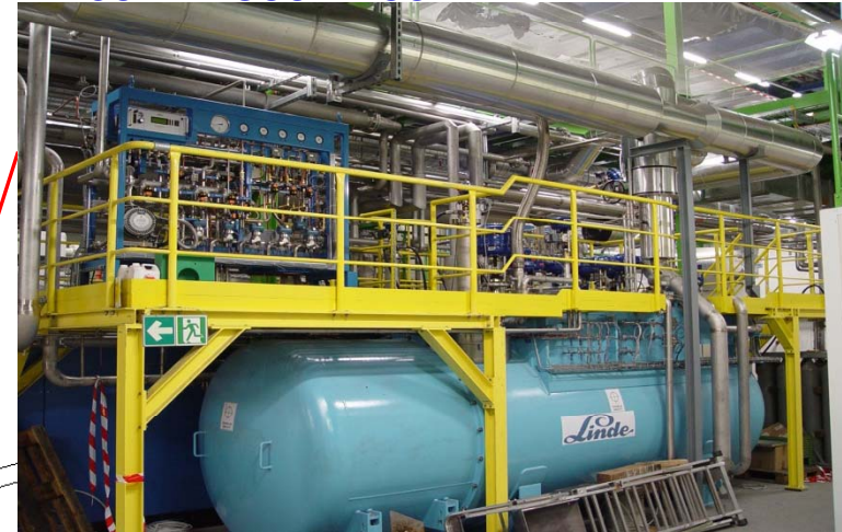
He Shield Refrigerator: - 20 kW 40 - 80 K - 60 kW 300 - 100 K
