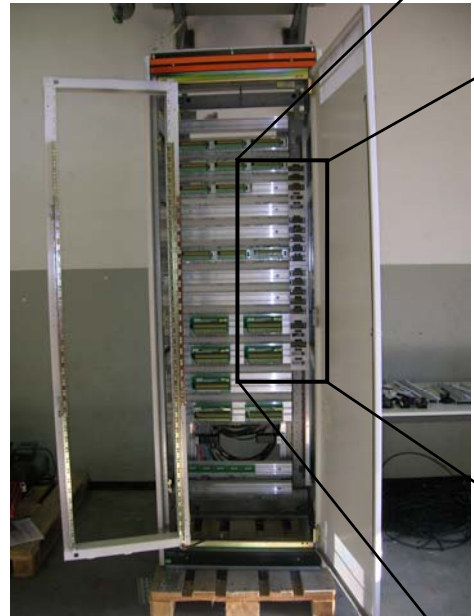
New PLC rack under construction
