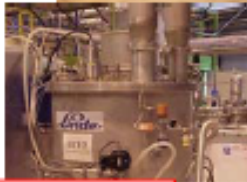
COLD COMPRESSOR (CC) The compressor pumps saturated helium at 3 K and at 10 mbar and compress it to 30 mbar.
