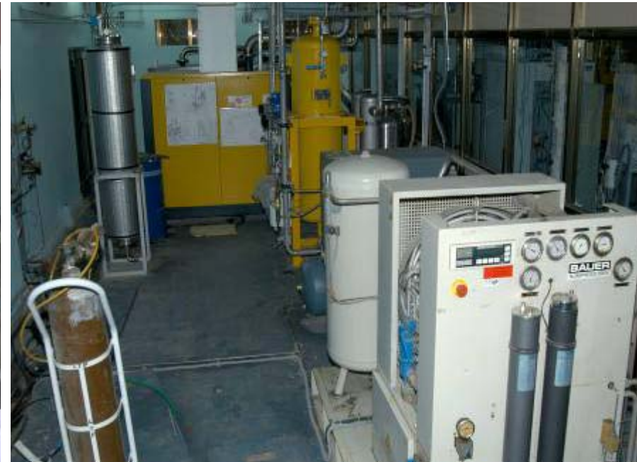
BAUER Model: G15.1, 22 m 3 /hr motor:11 KW
