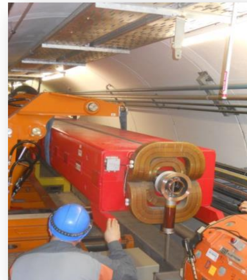
SPS magnet exchange
