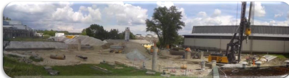
Installation of piles
