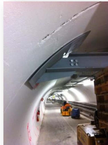
TT10 – vault repair
