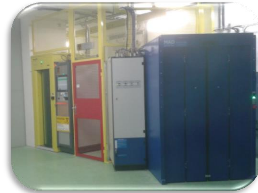
New PS access system
