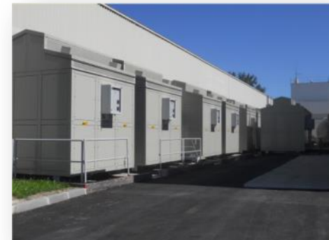
All new transformers in place
