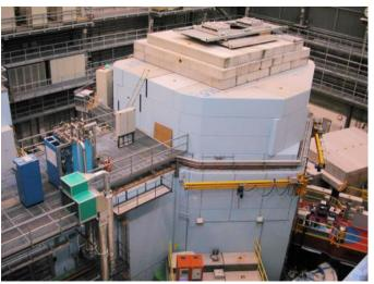
Target bulk shielding
