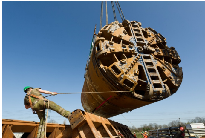
Removing the cutter head \varnothing 5.3m
