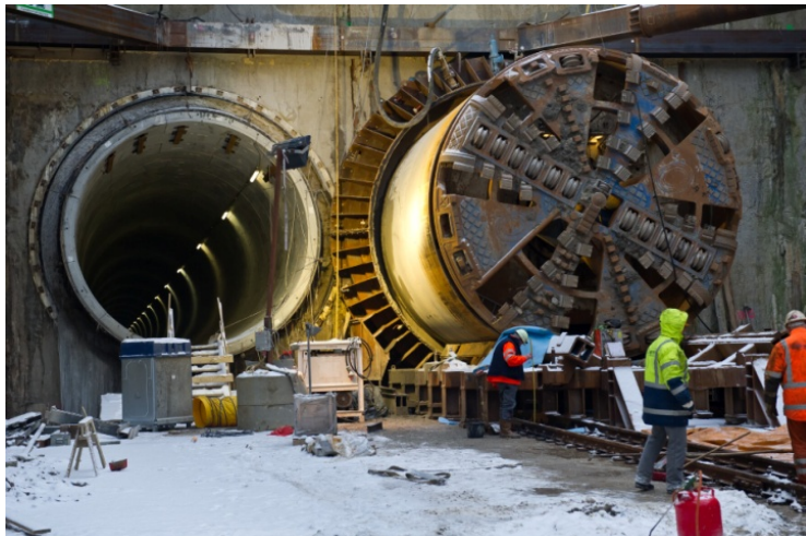
Breakthrough at beam switchyard
