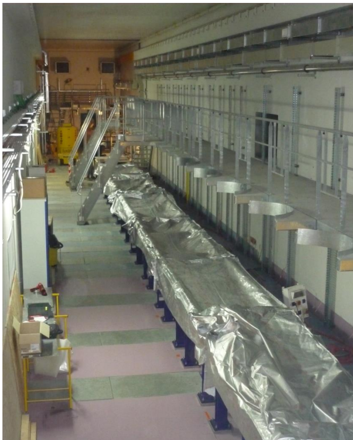
July 2013: mechanical frame in place
