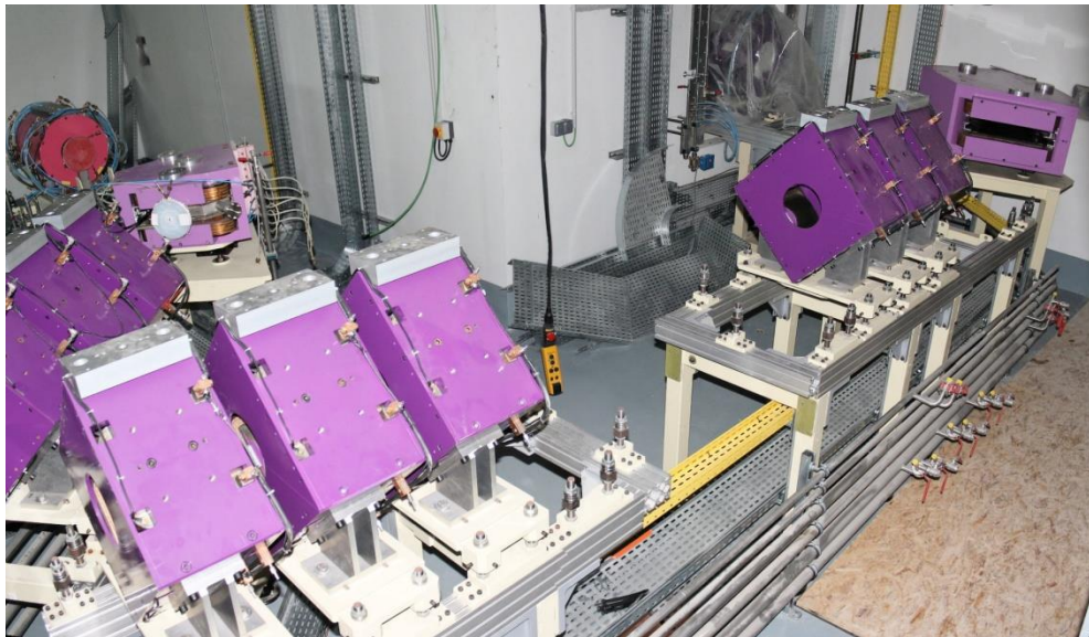
July 2013: mechanical frame and quadrupoles in place
