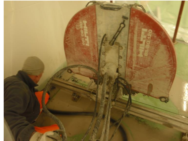
A trench cut for the cables
