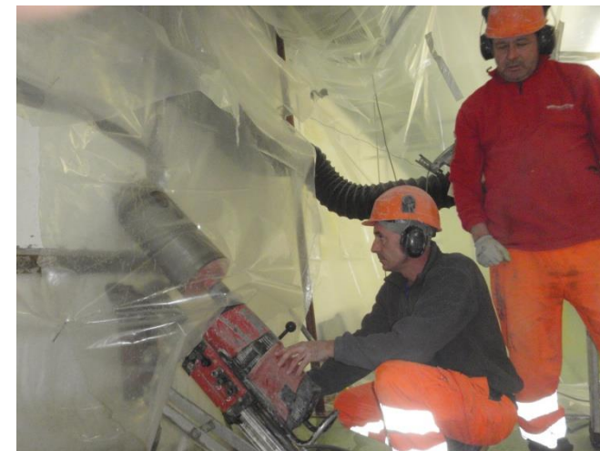
External wall drilled according to RP requirements
