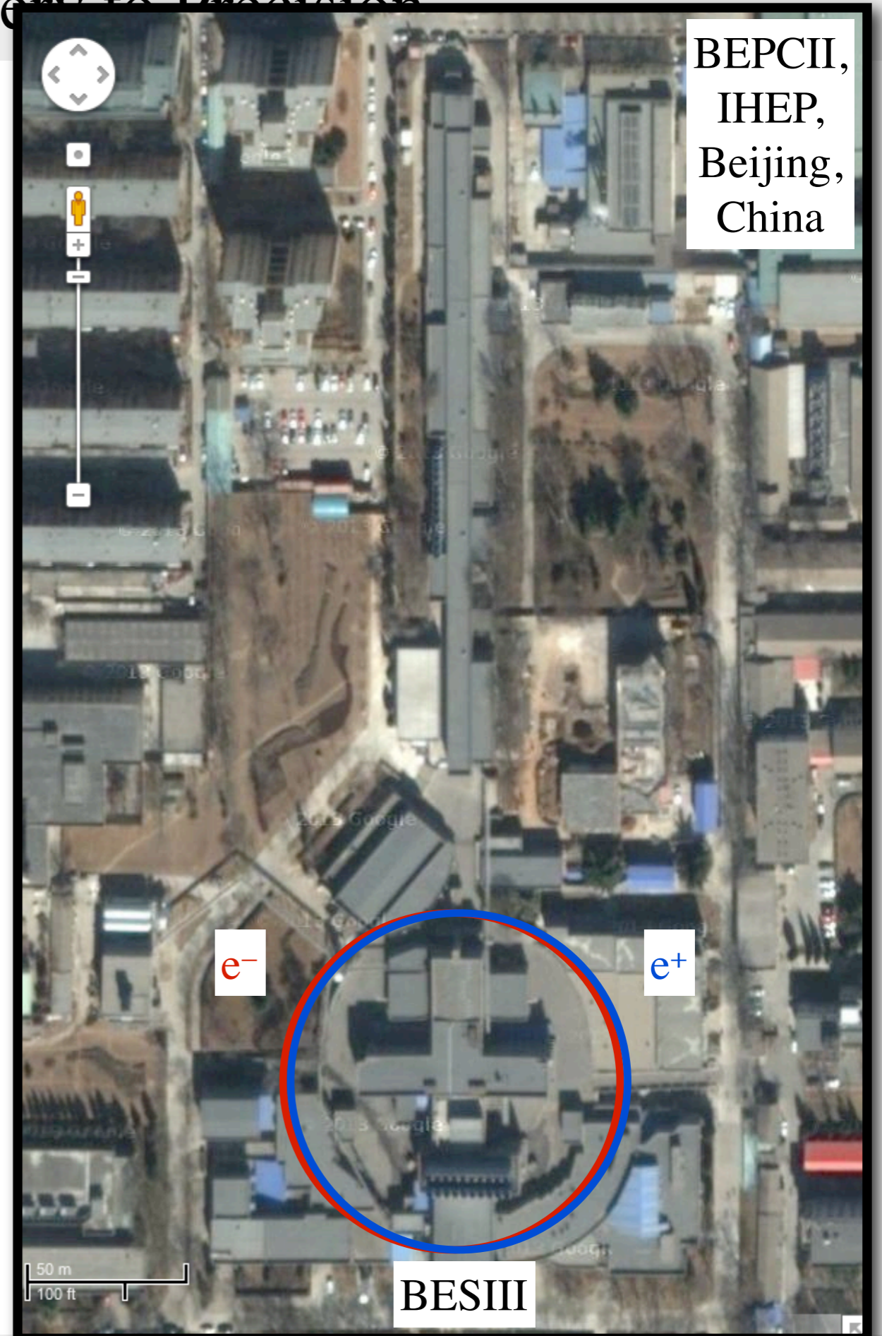
Google satellite image of BEPC-II
