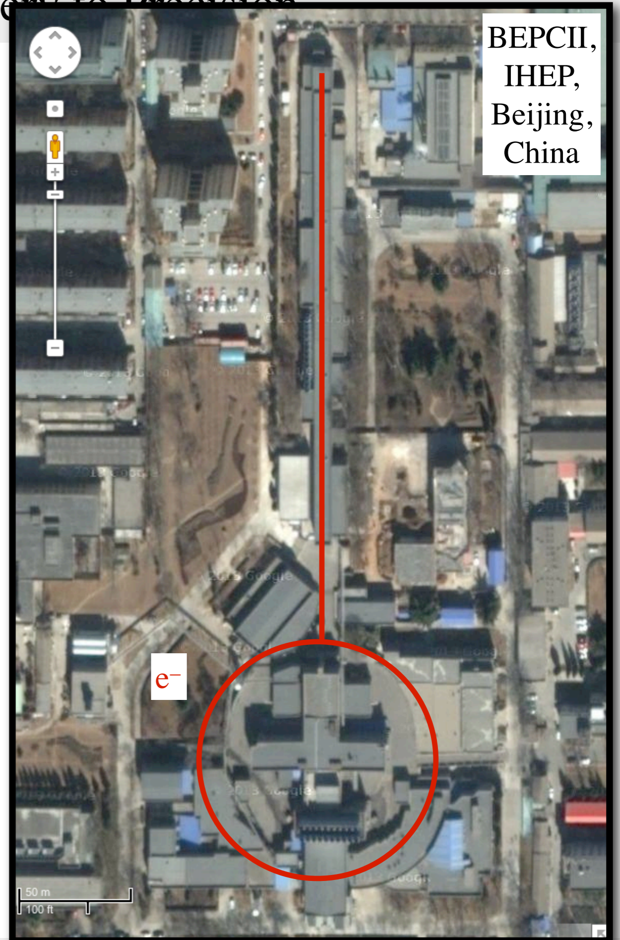
Google satellite image of BEPC-II
