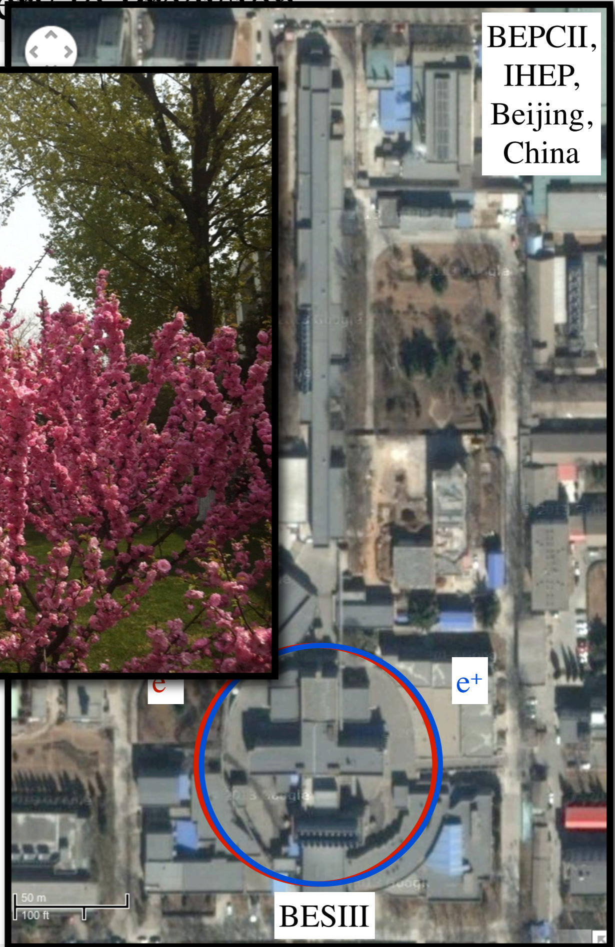
Google satellite image of BEPC-II
