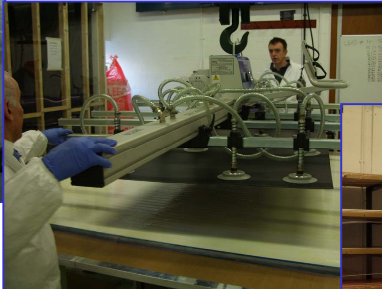
Lowering lead into position with vacuum-suction system
