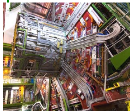
Multiservice cables (MSC) 43m + 5m + 0.5m (new)
