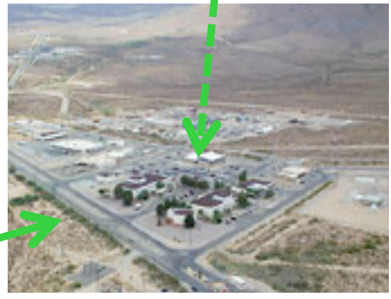
White Sands Ground Terminal, NM
