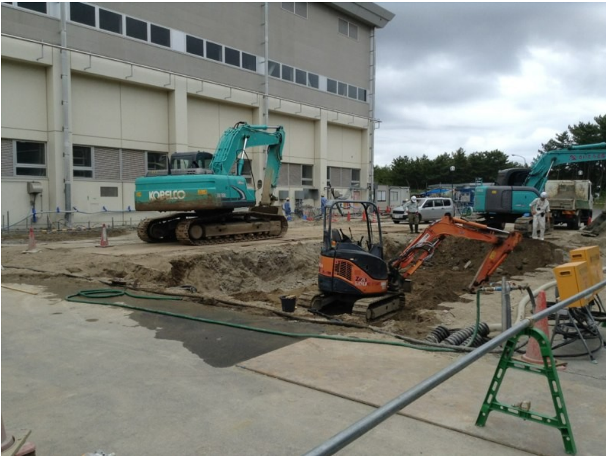
Excavation Started 4th June
