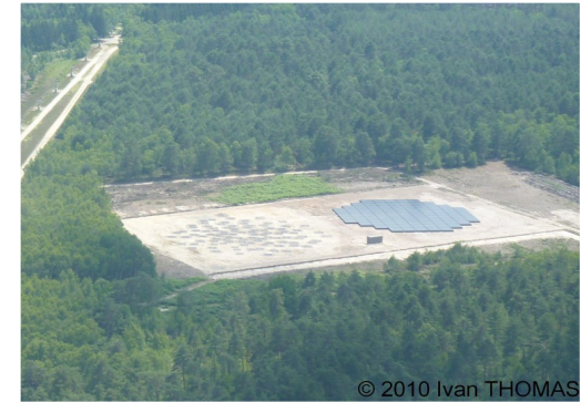
The LOFAR international station at Nançay – 192 antennas
