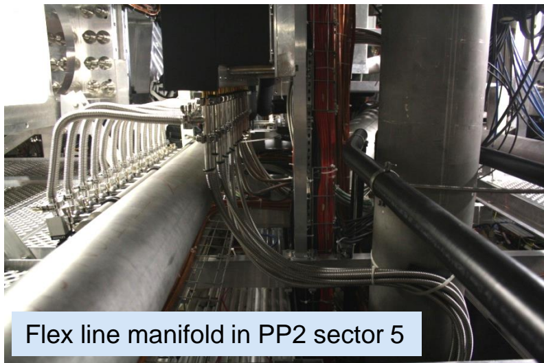
Almost identical: cooling lines and cables
