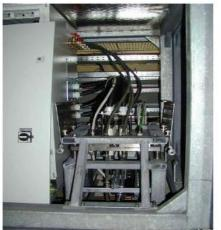
Power Supply Rack System with Docking → System for **fast replacement** of the entire unit
