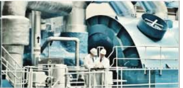
POWER GEN. & DISTRIBUTION
