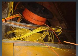
Excess fibres stored underneath the dipole behind the target. This is not what it was planned to look like!
