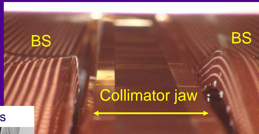
Damaged beam screen (BS) in a collimator
