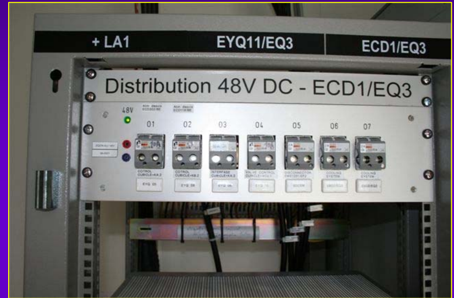
Distribution chassis with two independent sources, via diodes
