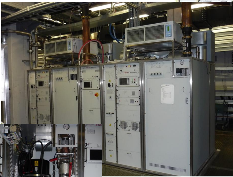
Elettra 500 MHz 150 kW IOT based amplifier for Combination of 2x80 kW
