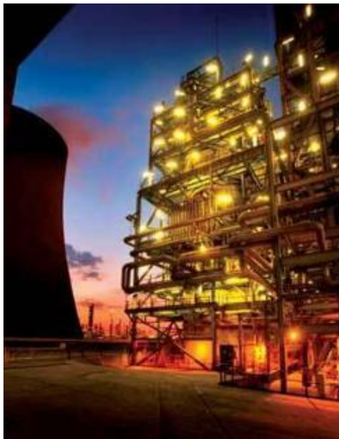
Sasol FT reactor at Secunda
