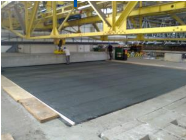
B151 PS BRIDGE AIR TIGHTNESS
