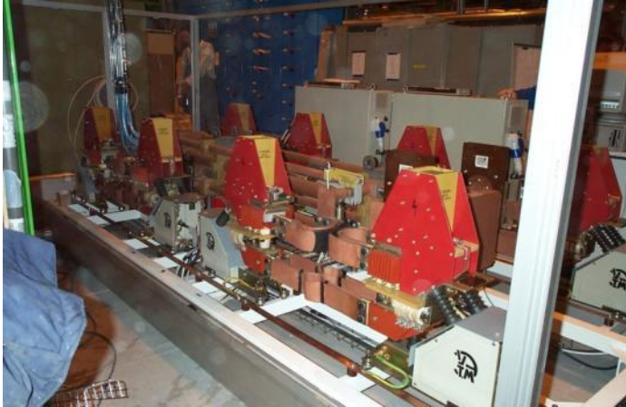
Assembly of 13 kA circuit breakers and dump resistors capable of dissipating 700 MJ.
