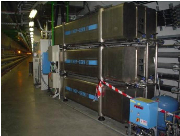
Assembly of 13 kA circuit breakers and dump resistors capable of dissipating 700 MJ.
