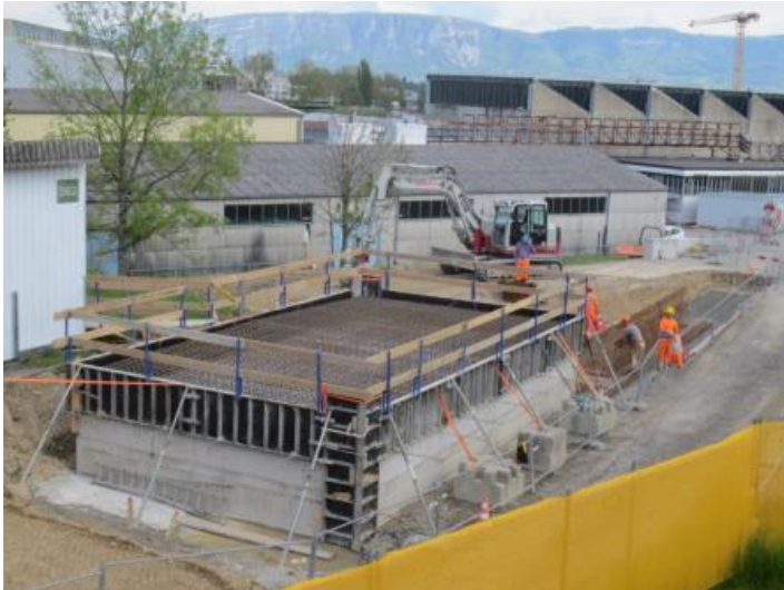
Extraction region shielding increase (above SS16)
