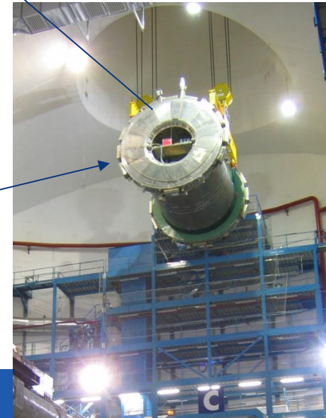
Liquid argon barrel calorimeter cryostat during lowering in the pit
