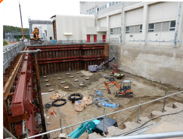
Construction of COMET experimental hall.
