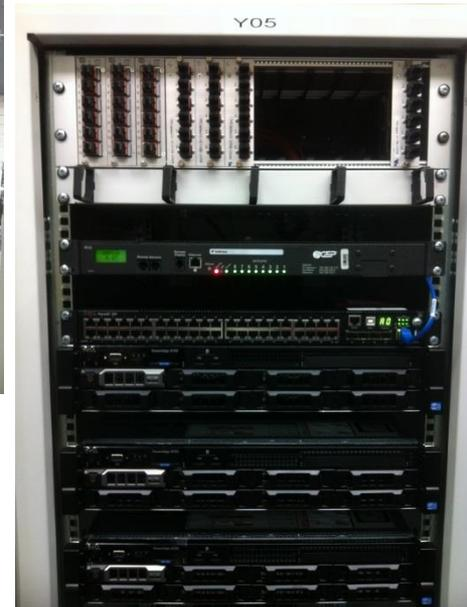
DAQ in CR1 being reinstalled after full replacement and extension of hardware.
