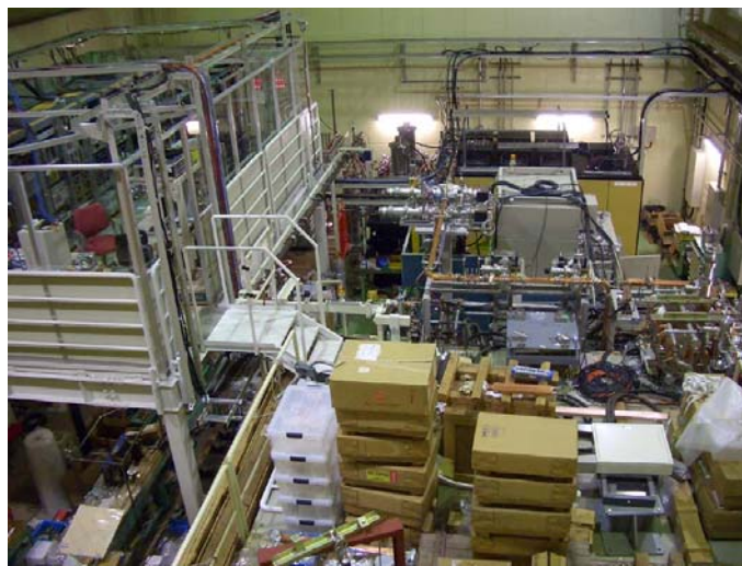
Two klystron facility
