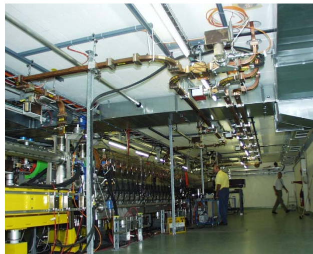
In CLEX tunnel
