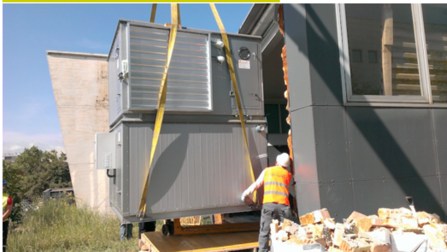
Installation of free-cooling units
