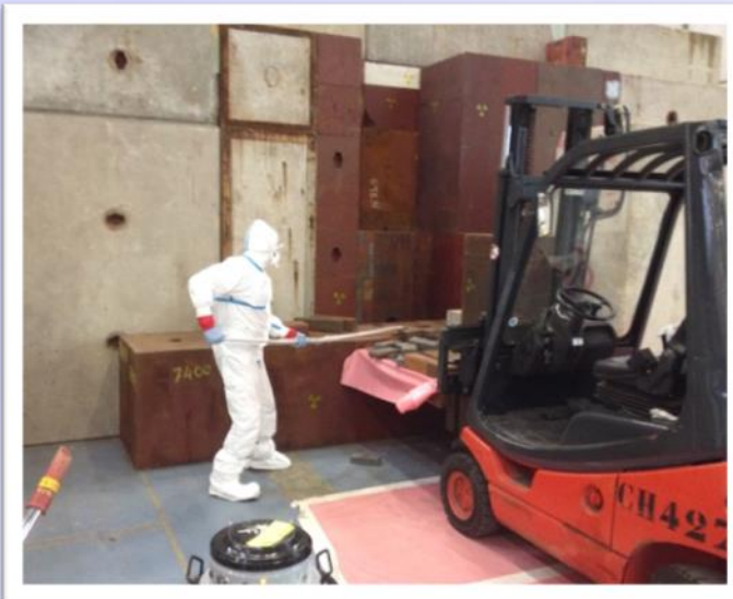
Handling of most radioactive Pb/Fe bricks with dedicated tool
