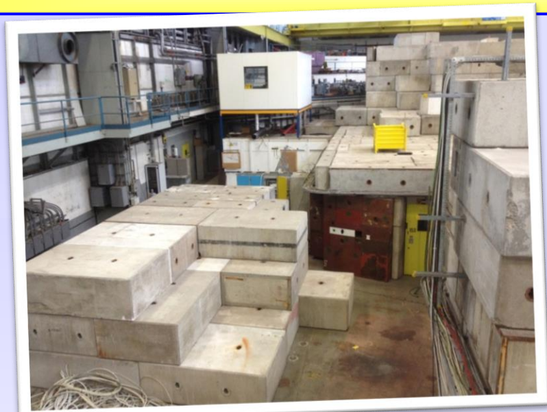
T7b area dismantled
