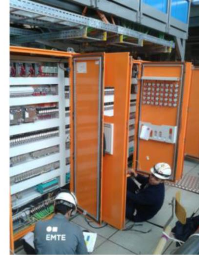
CV cabling works
