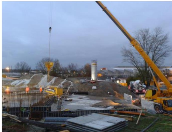
Septum 16 shielding - formworks
