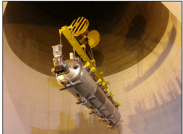
Figure 1: The spare RF cryomodule (four cavities) being lowered down into the UX45 cavern (Feb. 2014).
