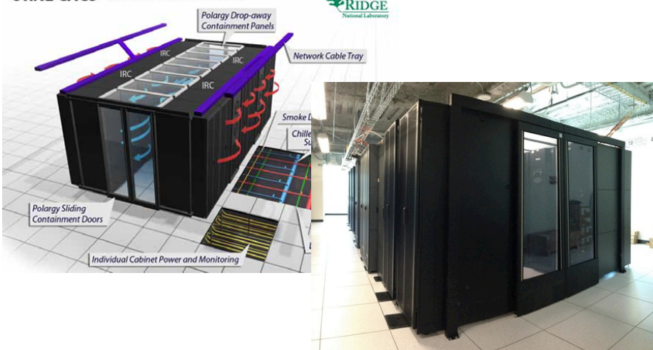
ORNL CACS - Cold Aisle Containment System
